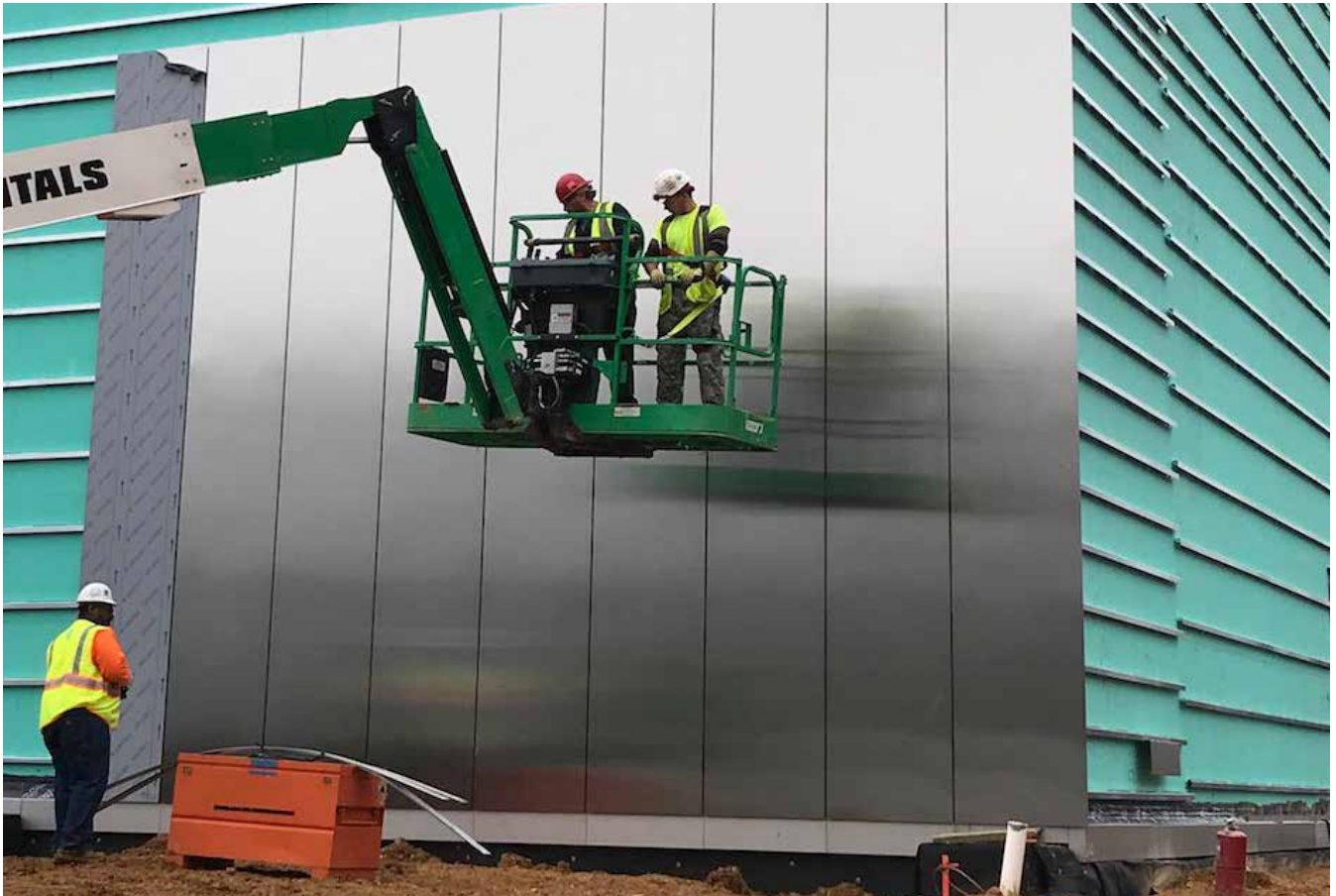
Stainless Steel Panels start to go up-February 2018
